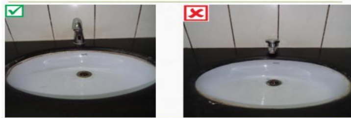
Figure 19: Touch free (hands free) taps at wash basins to
