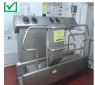
Figure 23: Automatic hand-washing and foot cleaning system
