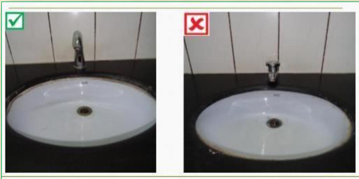
Fig: Touch free (hands free) taps at wash basins to avoid cross contamination
